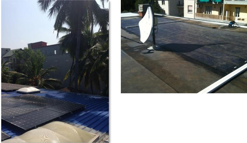
**Fig. 2:** small shading, big losses: evidence of poor design in (a) Lagos, 2016, and (b) Italy, 2009.
